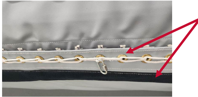
Figure 19: Samples of hardware and components to inspect
