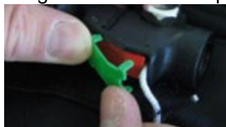
Figure 27 - Installing the green indicator clip
