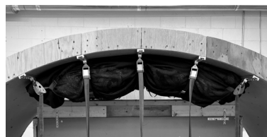
17.8 Tighten both corner straps 89102-002 as much as possible (they should have further to go).
