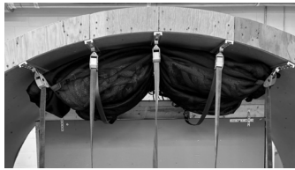
17.5 Tighten both corner straps 89102-002 as far as they will go.
