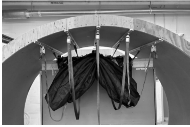
17.1 Tighten center strap 89102-004 halfway.
