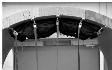
17.7 Tighten the center strap 89102-004 as much as possible.
